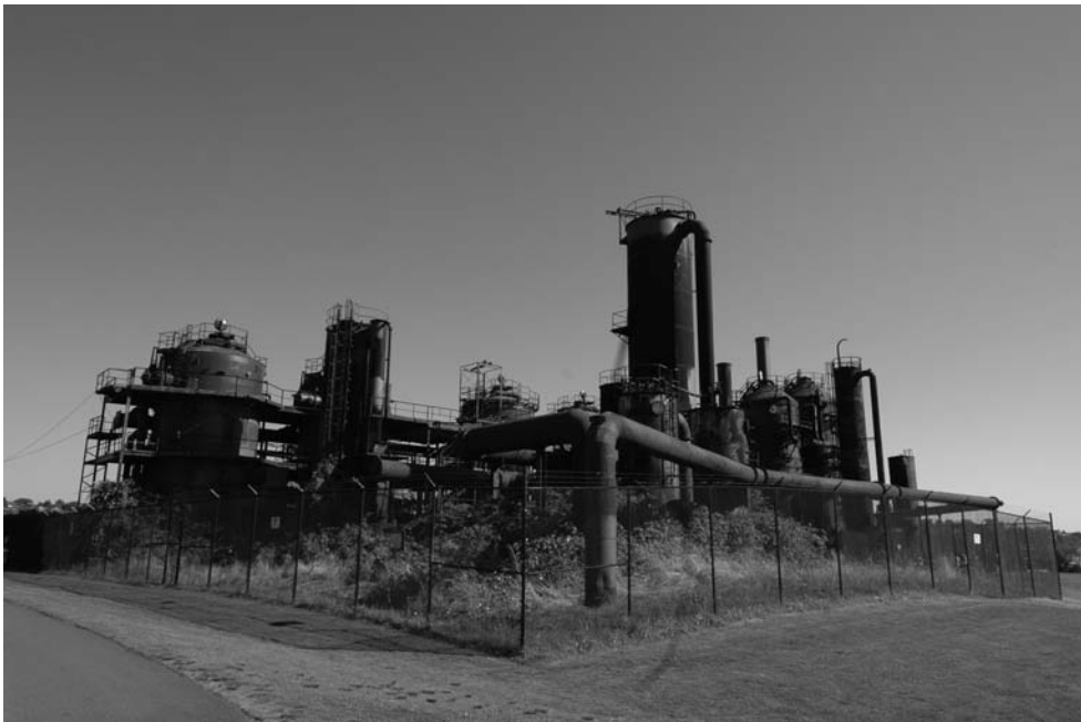
Figure 34.3 The fenced-in industrial relics at the Seattle Gas Works Park. (source: Daniel Winterbottom)
